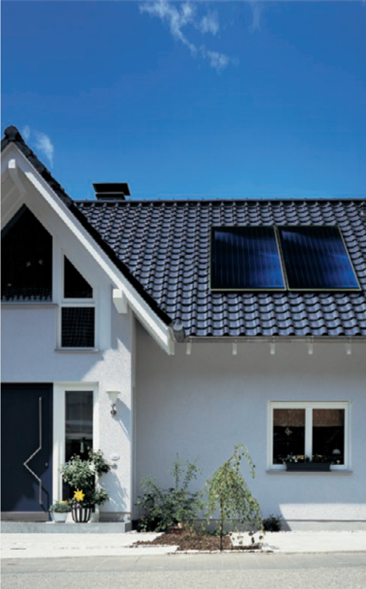
Environmentally friendly solar energy for heating water and for supporting the central heating system
